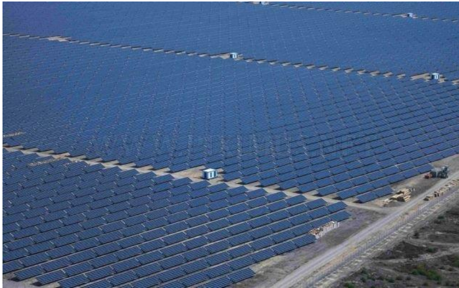
Lieberose 71 MegaWatt (electric) Solar Power Plant near Berlin in Germany
